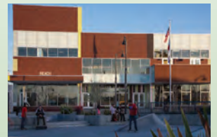
REACH Ashland Youth Center is LEED® Platinum certified.
