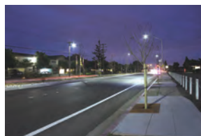
7000 streetlights were retrofitted with LEDs.
