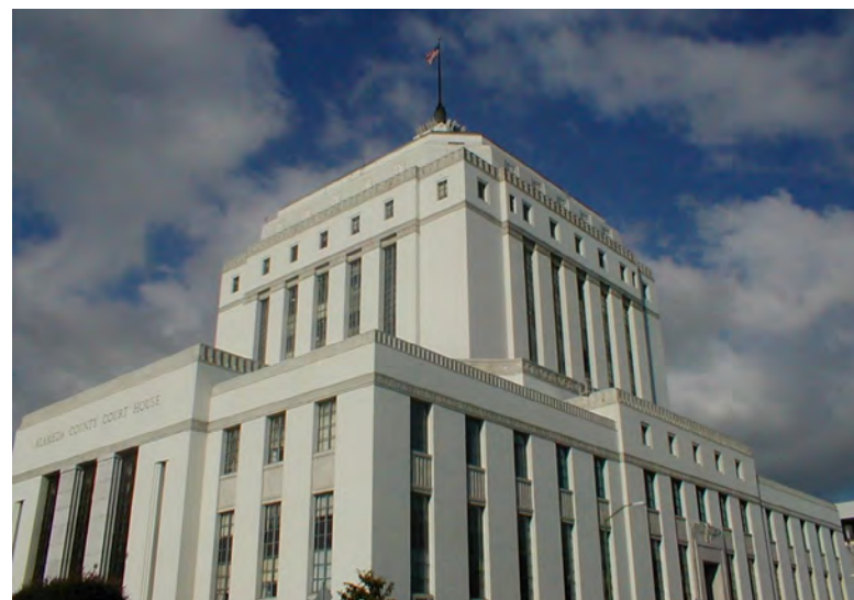
The René C. Davidson Courthouse, completed in 1934, is one of the oldest buildings the County maintains in our portfolio.
