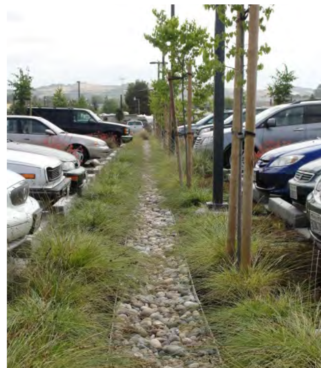
A bioswale in Castro Valley Library parking lot channels stormwater to remove pollution, reduce runoff, and allow water to absorb into the ground.
