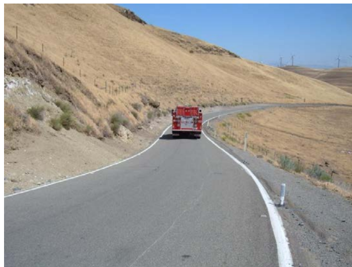
Patterson Pass Road in the Vicinity of Mile Marker 6.4: narrow roadway width.
