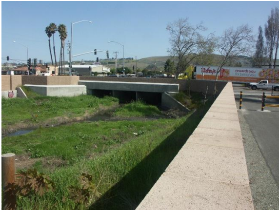
Photo 1: Phase I floodwall looking northeast (upstream) towards Huntwood Avenue.
