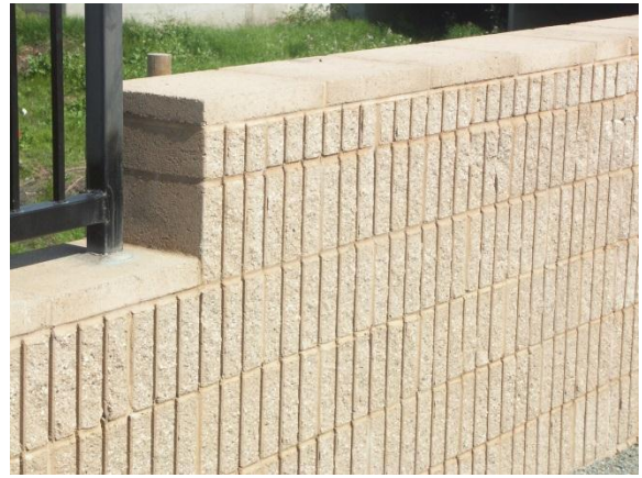
Photo 2: Close-up of Existing (Phase I) floodwall.
