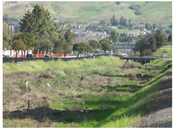
Photo 4: Phase II, proposed project site, looking northeast (upstream) towards Union Pacific railroad crossing.
