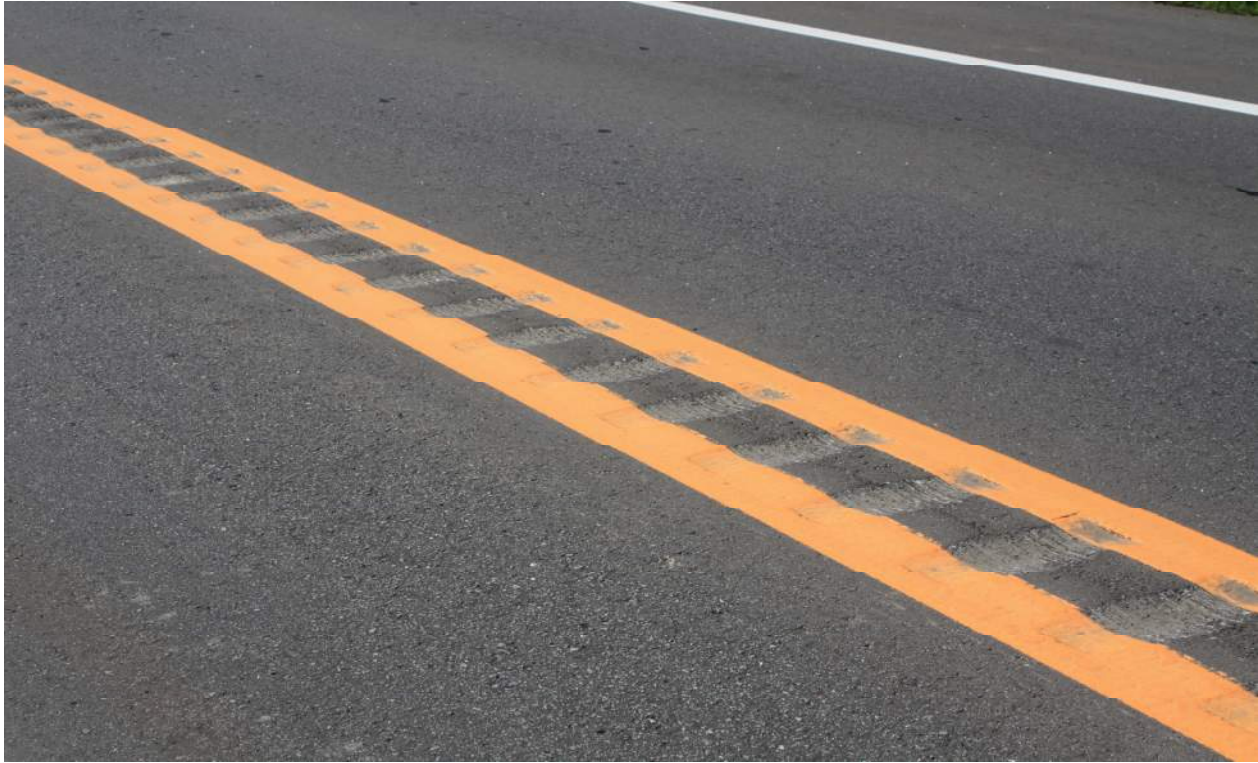
Figure 18 Typical Centerline Rumble Strip
