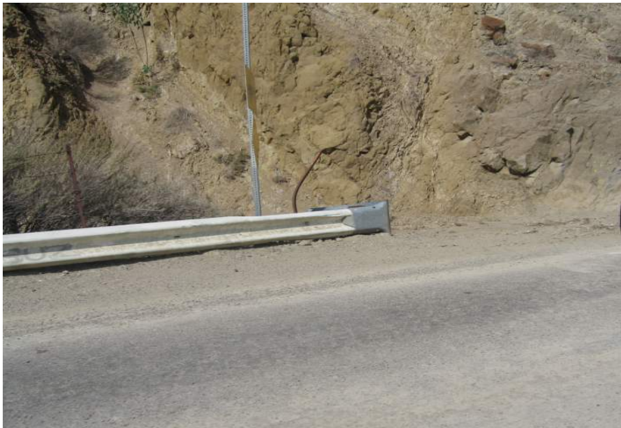
Figure 4 Guard rail with non-standard height
