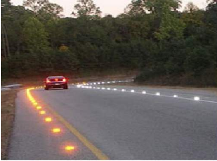
Figure 14 Reflective Pavement Markers
