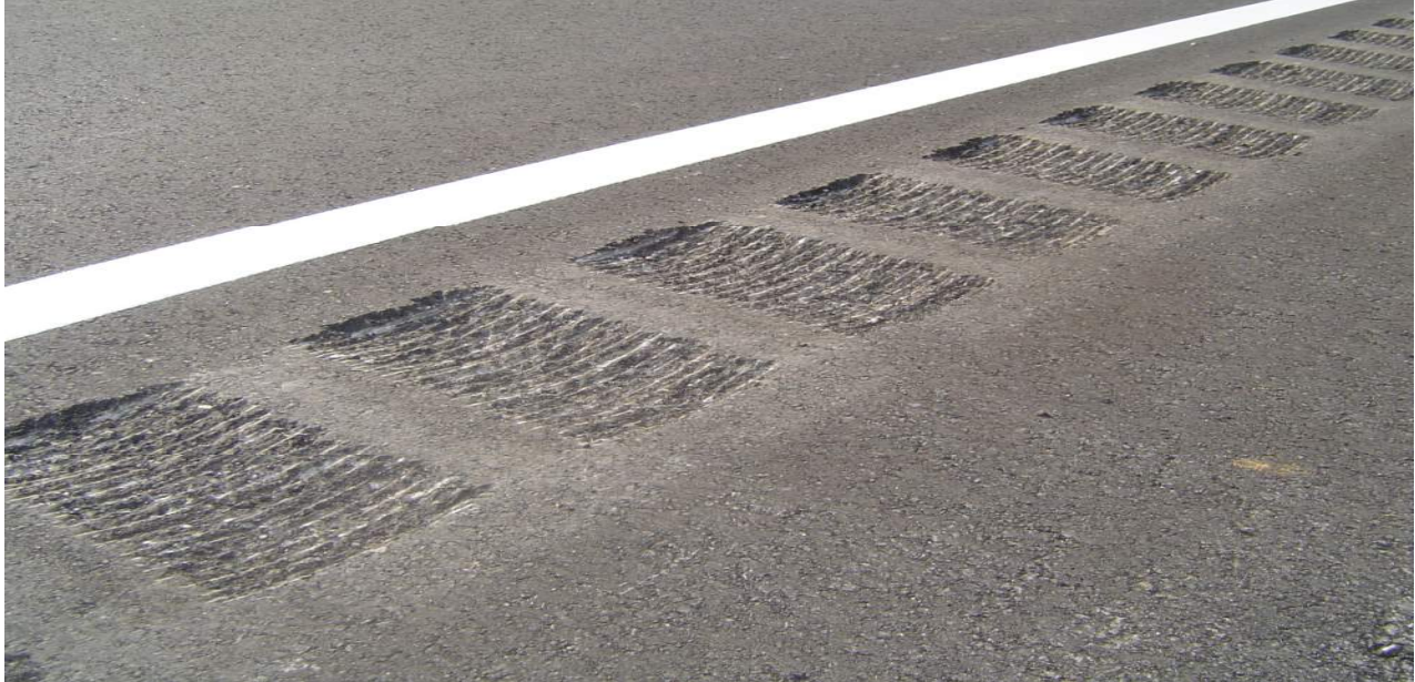
Figure 19 Typical Shoulder Rumble Strip
