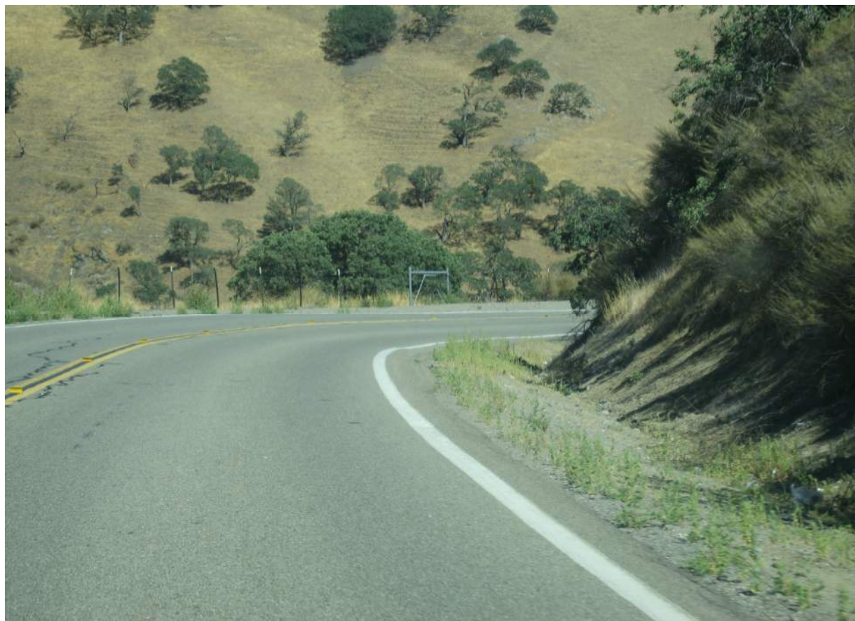
Figure 2 Typical horizontal curve with limited sight distance on Tesla Road
