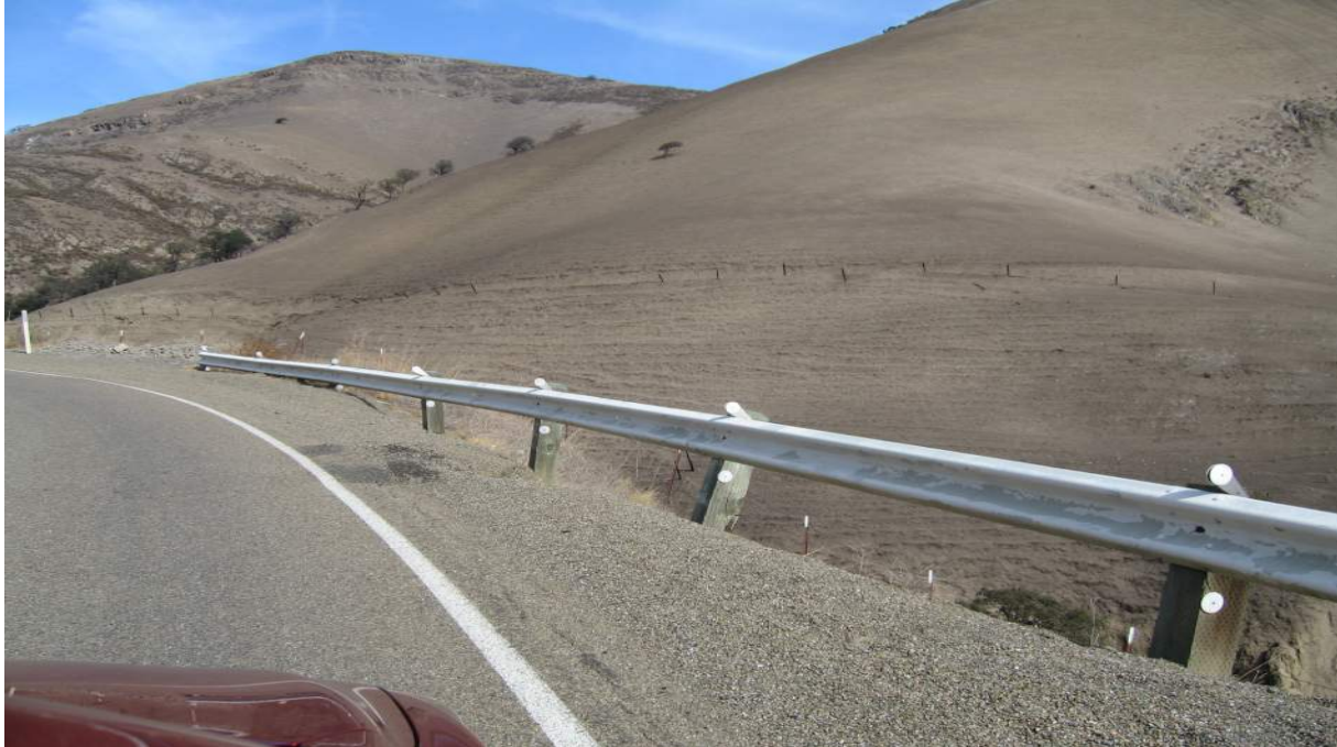
Figure 20 Example of guardrail replacement that requires re-grading of embankment
