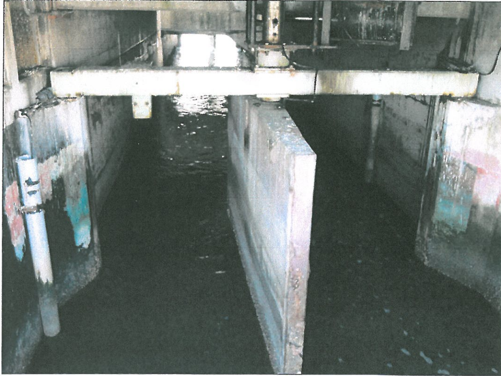
GS-1 Gate and Suction Channel Typical Location of Gate Graphite Anodes
