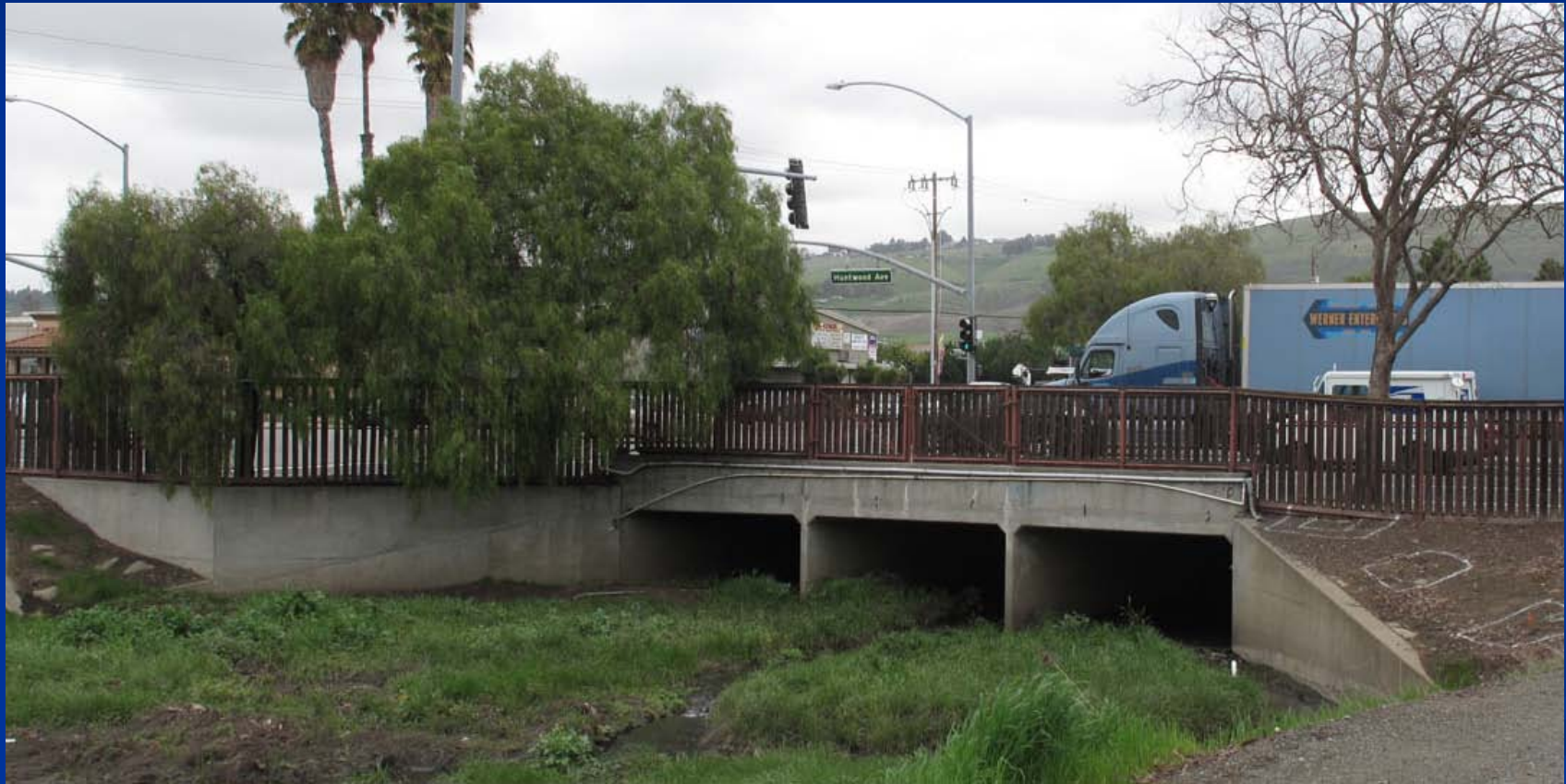
Huntwood Headwall Existing view from inside the channel
