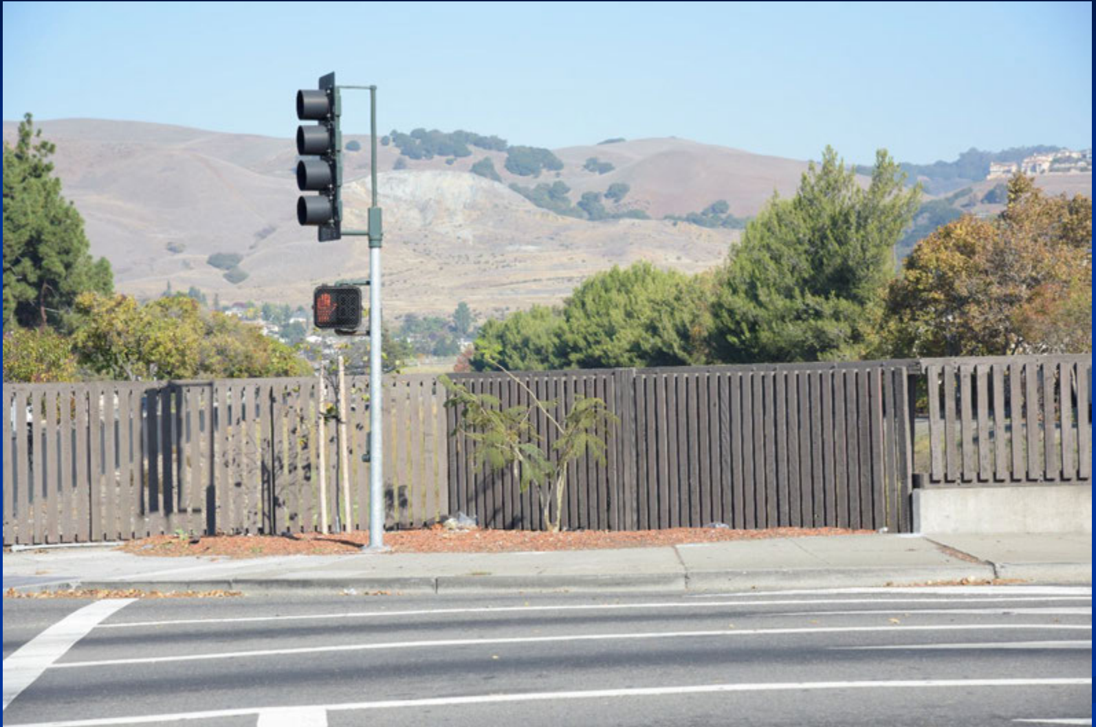
Street View Huntwood Headwall - Phase II
