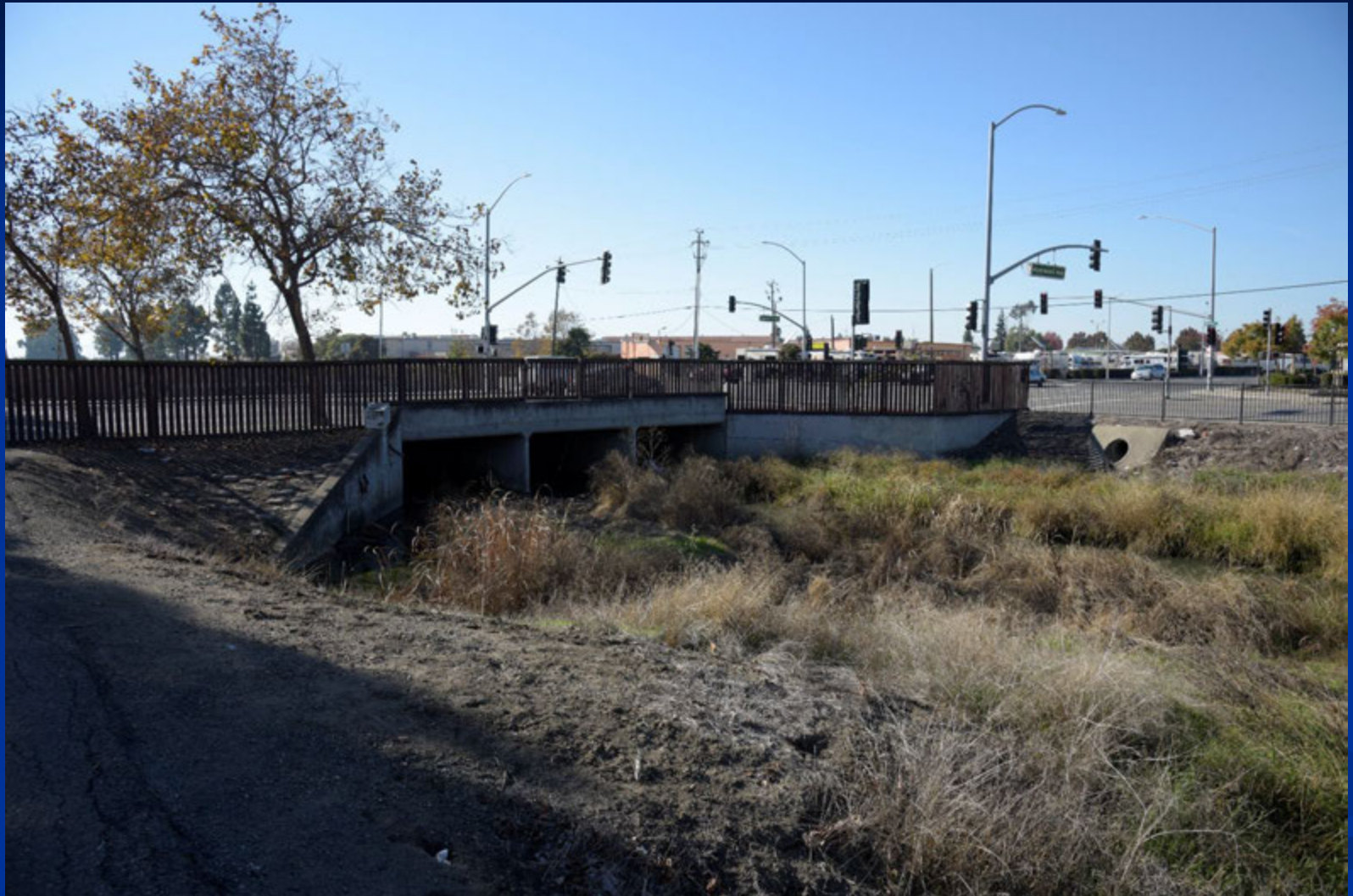
Existing Huntwood Headwall from inside the channel
