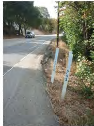
Photo 2. Sheet Flow to Roadside Ditch (PM 5.83, Lt)
