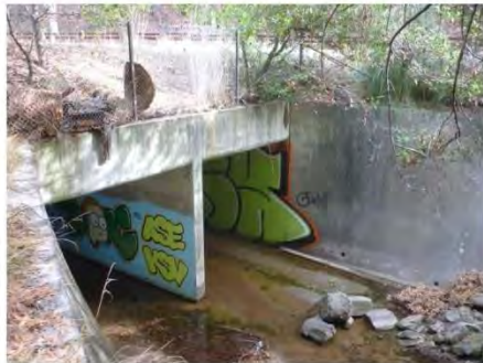
Photo 5. Box Culvert for Crow Creek (PM 1.66, Lt)
