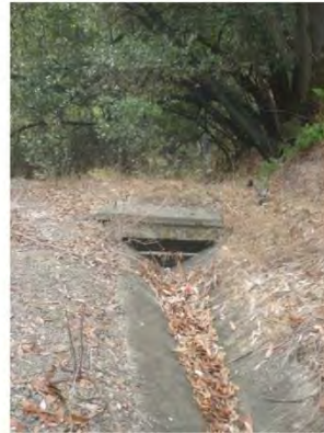
Photo 4. Lined Ditch to Drop Inlet (PM 1.66, Lt)
