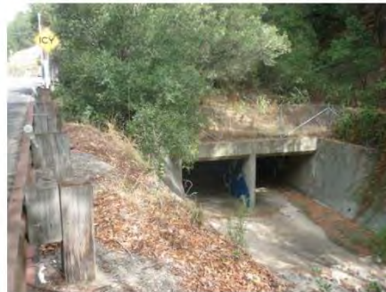
Photo 6. Box Culvert for Crow Creek (PM 1.96, Rt)
