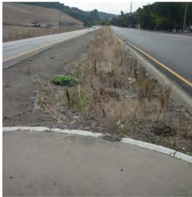
Photo 3. Ditch at Median (PM 3.85)
