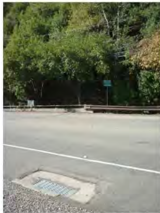
Photo 1. Curb and Inlet (PM 1.30, Rt)
