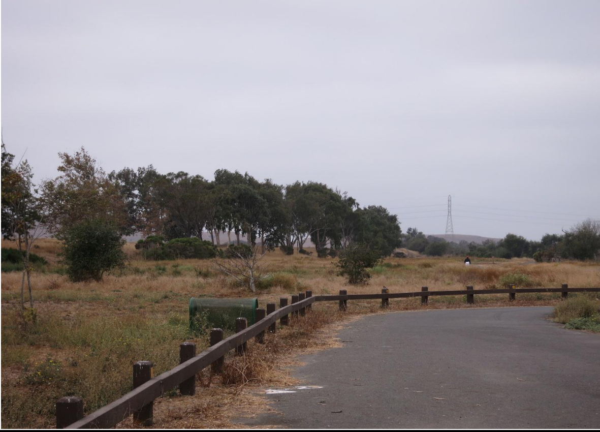
Photo 1: View of North Levee Looking West from Parking Area
