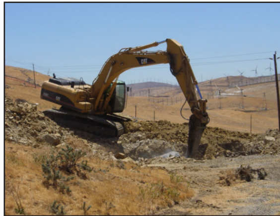
Breaking up the foundation
