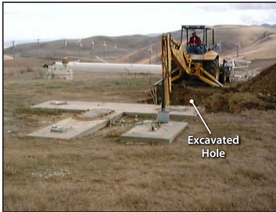
Excavation of hole adjacent to foundation
