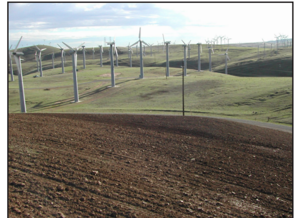
Area has been graded and seeded
