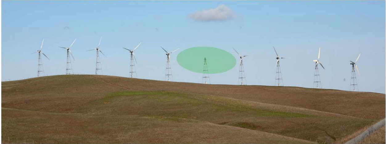
Photo 5. Turbine relocations would be relatively safer at towers interior to the turbine rows and atop a hill or ridge.
