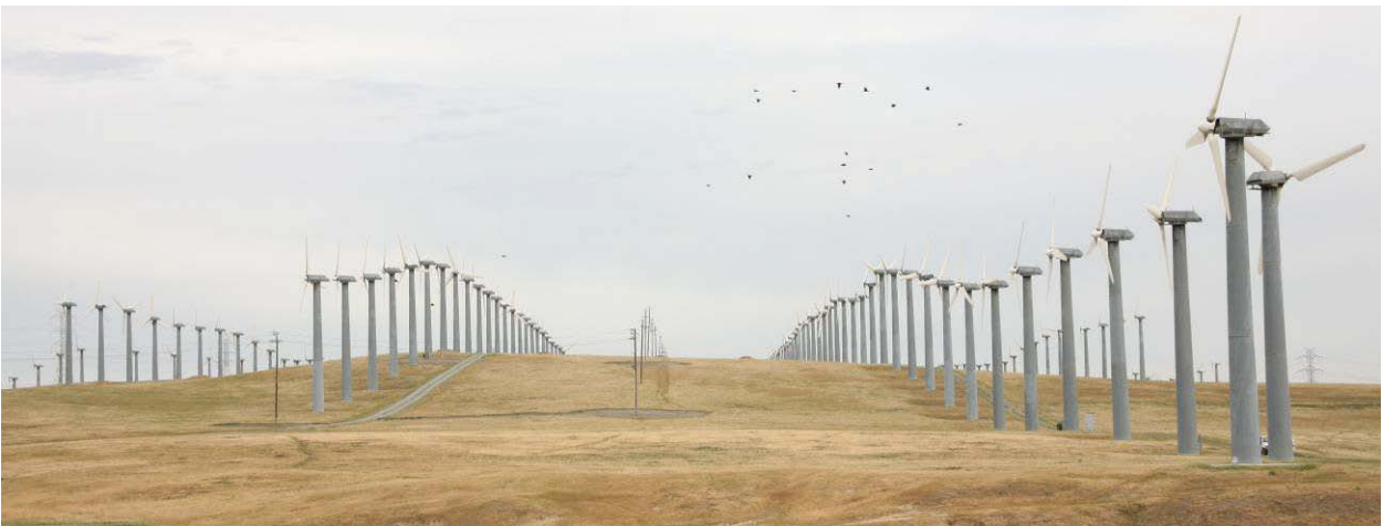
Photo 4. Where possible, turbine relocations should be directed to the interior aspect of relatively denser turbine fields.
