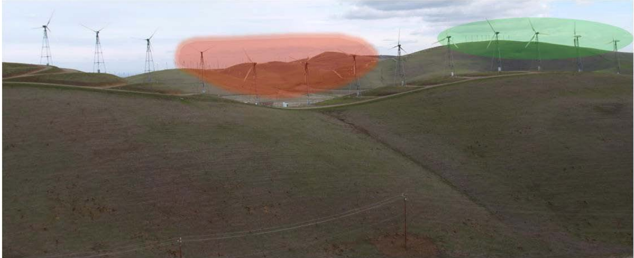
Photo 9. Turbines should be relocated to hill peaks or ridge crests (e.g., green highlight), but not to saddles in the ridge (red highlight).
