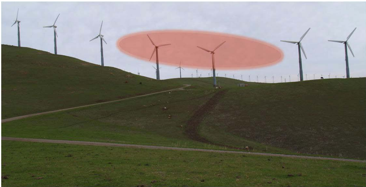
Photo 15. Wind turbines should not be relocated to shoulders of the ridge or hill, or where the slope suddenly changes, such as seen in this photo.
