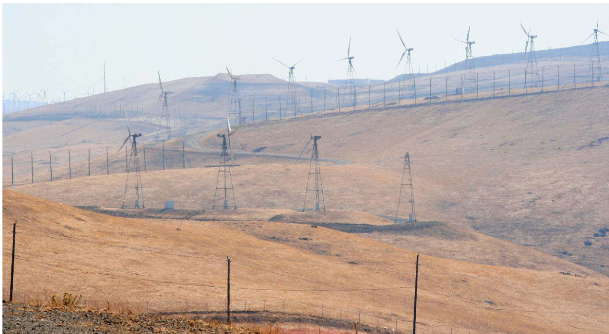
Photo 8. Turbines should not be relocated to ends of turbine rows, especially where the towers are next to steep slopes or ravines, such as the derelict tower on the right side of the turbine row in the foreground.
