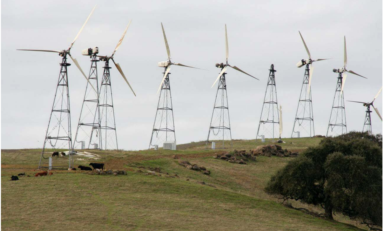
Photo 18. Derelict towers should not be put back into service where they occur near rock piles or trees or other structures that may be attractive for perching or hunting. In the photo above, rock piles appear just this side of the derelict tower, which should be removed. Note, however, that removing the derelict tower would result in a potentially hazardous gap in the turbine string, suggesting the importance of fully evaluating all hazardous conditions before a relocation or removal decision is made.
