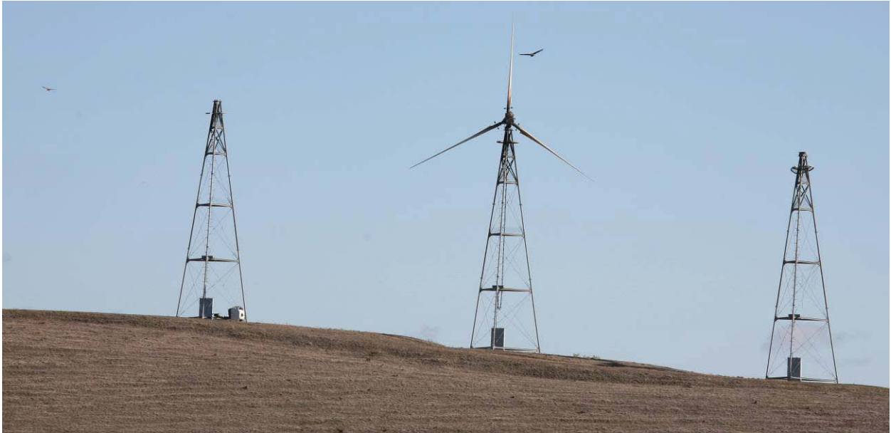
Photo 1. The two derelict towers to either side of this functional turbine on the ridge crest should either be removed or put back into service. If the derelict towers are removed, then the interior functional turbine should also be removed.
