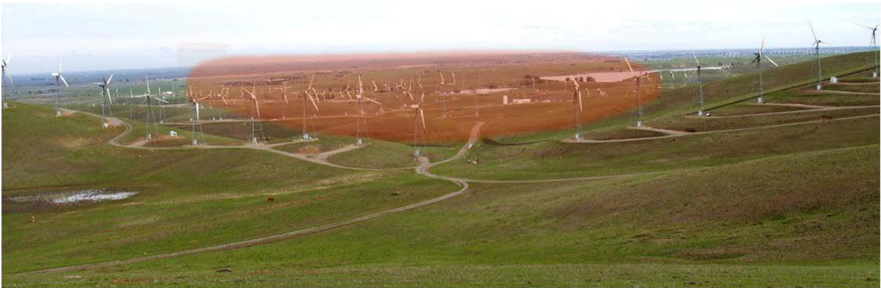
Photo 12. Wind turbines should not be relocated to saddles formed by the meeting of two ridges.
