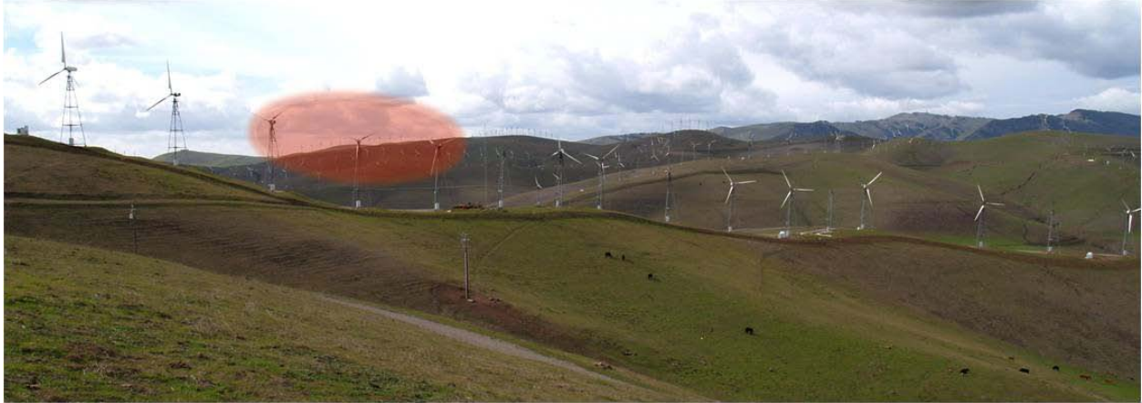
Photo 16. Wind turbines should not be relocated to shoulders of the ridge or hill, or where the slope suddenly changes, such as seen in this photo. This is especially true for long turbine rows like this one, where opportunities for raptors to fly through gaps are absent.
