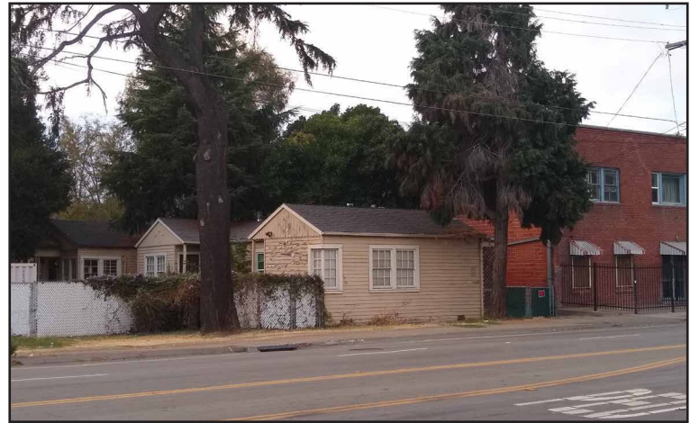
Looking north from A Street, project site on left (single-story building to be demolished) and warehouse on right
