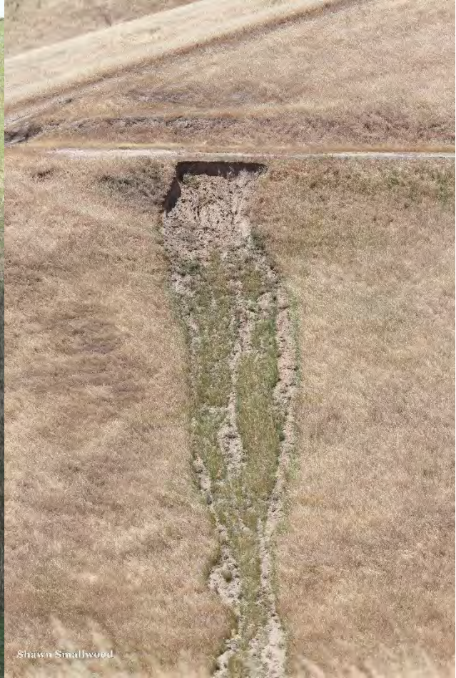
Photos 14 and 15. Beginning with construction and continuing through project life, soil erosion originates from access roads, turbine pads, and pipe culverts throughout the APWRA.
