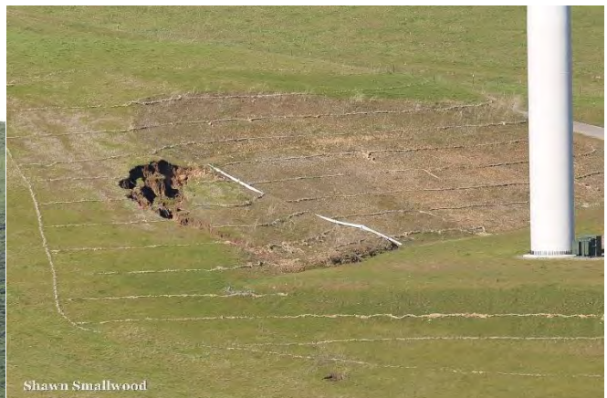
Photos 16 and 17. Soil origin in wind projects often originate at the corners of turbine pads (left) or on cut slopes (right).
