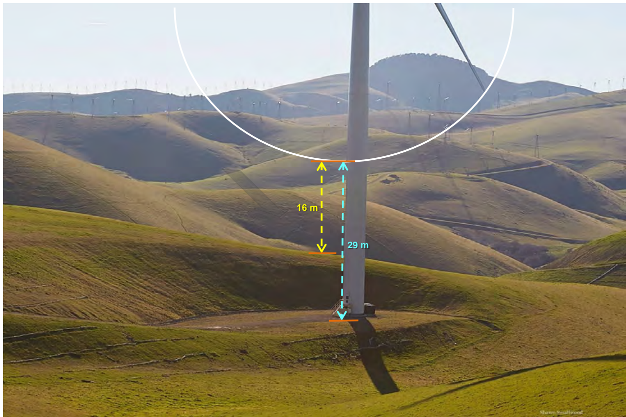
Photo 18. This view is toward the prevailing wind (see broad, semi-transparent, white arrow), so the prevailing upwind slope, the crest of which is only 30 m from the wind turbine, forces any bird or bat passing over it into a vertical gap of only 16 m between the hill crest and the low reach of the blade . The wind turbine's 29 m ground clearance of the low reach of its blade-sweeps is no longer the clearance experienced by birds and bats. This turbine became the most prolific killer of red-tailed hawks in the project.
