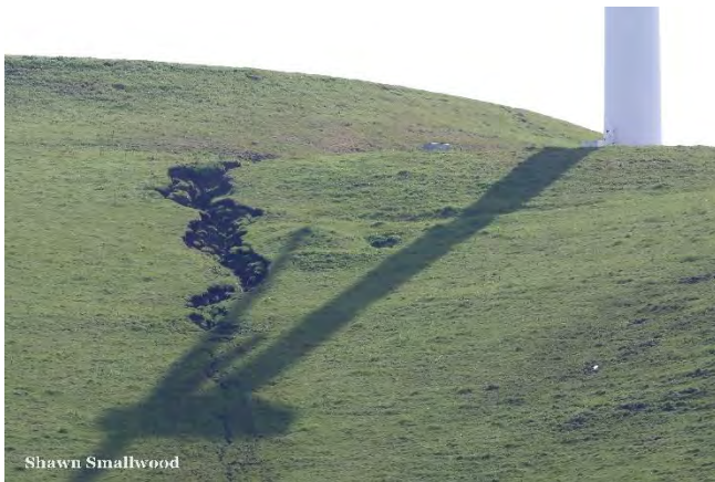
Photos 16 and 17. Soil origin in wind projects often originate at the corners of turbine pads (left) or on cut slopes (right).
