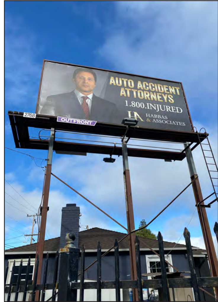
South billboard located at 970 East Lewelling Boulevard (APN 414-6-46).
