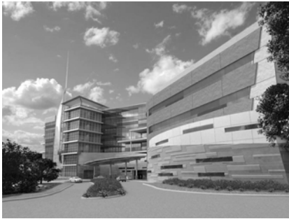
The existing hospital building (top picture) will be demolished following completion of the new Eden Medical Center Castro Valley Facility.
