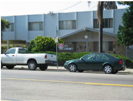
Apartment complex in the Eden Area
