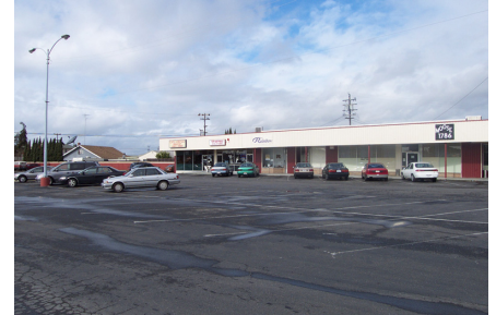
Shopping center on Bockman Road
